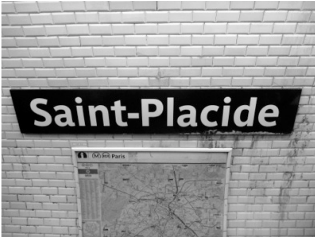
Figure 4. Mold on a signboard
